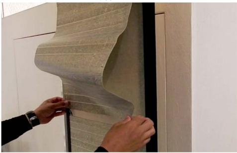
•Roll each seam lightly with a seam roller. Do not to roll too hard. (Set the both edges perfectly for butt joint.)
