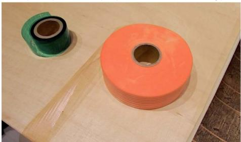
•Put plastic protective strip on the top of lower wallpaper backside.
