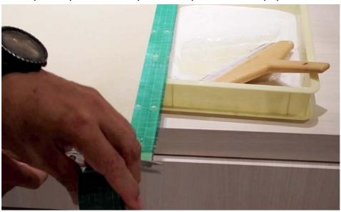
• Put plastic protective strip on the bottom of upper wallpaper backside, where overlaps.
